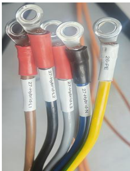
Figure 7- 14 Auxiliary power cable for Cabinet
