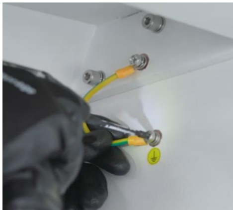
Figure 7-9 connect the ground cable of sunshade to cabinet enclosure
