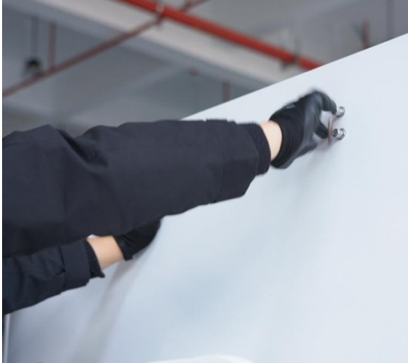
Figure 7-7 remove the pre-installed bolts from the cabinet enclosure
