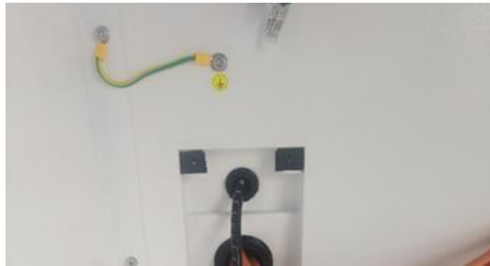
Figure 7-35 Panel ground cable installation
