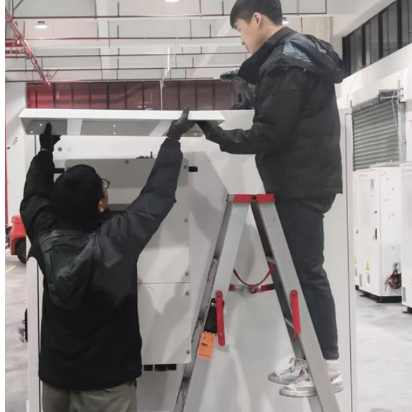
Figure 7-8 fixing the sunshade to cabinet enclosure
